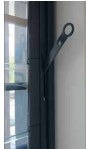
Ringpull handle for out of reach louvre placement
